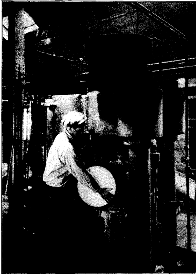
FIGURE 73. Smokeless Powder Manufacture. (Courtesy E. I. du Pont de Nemours and Company, Inc.) Dehydrating Press. The nitrocellulose comes from the dehydrating press in the form of a cylindrical block, impregnated with alcohol, ready for the mixer where ether is added and where it is colloid.
